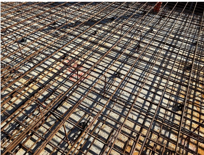
Figure 1: Transmutation Bar Chairs in MFRO slab
